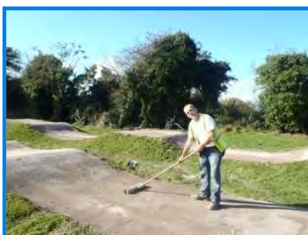
Repaired Track at the Rec.
